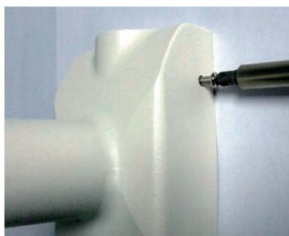
10. Secure bracket onto plate with 2pcs of M4xL10 screws.
